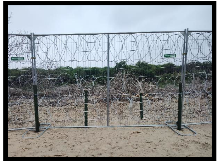
View of deterrent fencing along Rio Grande in project area
